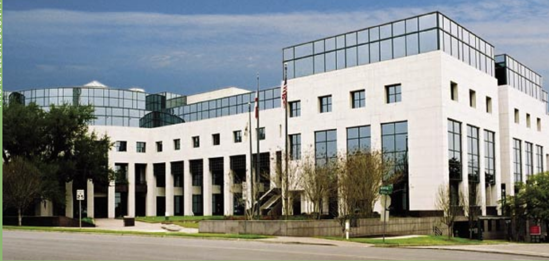
PHOTO: LEON COUNTY
