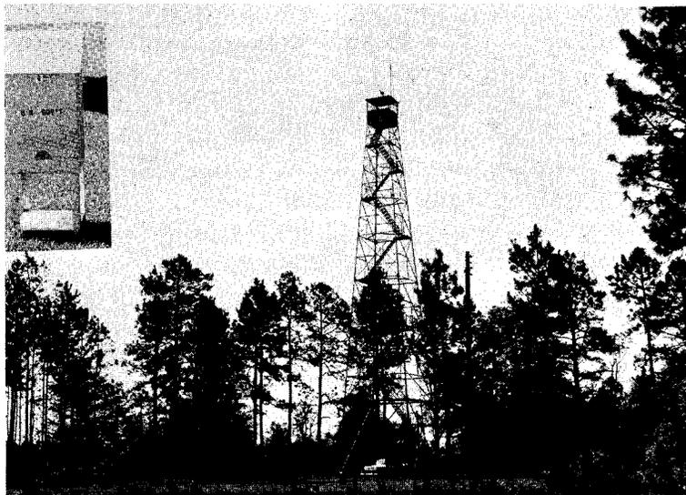
FIG. 2. A typical Georgia Forestry Commission fire lookout tower with one high-volume air sampler located on the second landing below the cab and the other one at the base of the tower.
